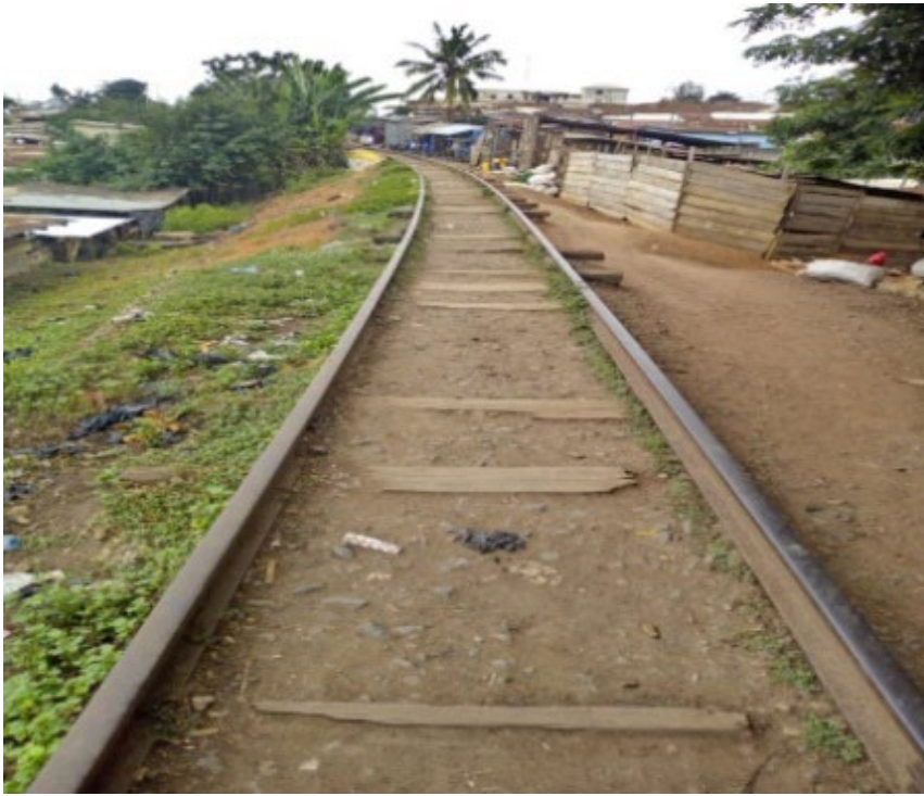
Fig. 2.12: Railway line at Oforikrom
